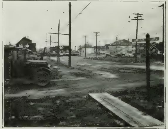
Fog at Oak Street and Fifteenth Avenue. Recommended for Improvement.
